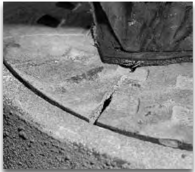
Close-up of the 9" x 9" load block rubber pad lid and frame with the lid broken from proof load testing.
